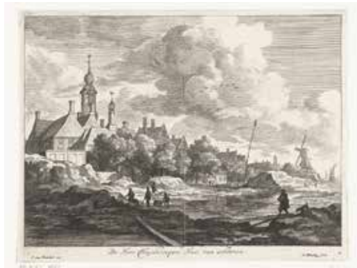
Fig. 10 Abraham Bloteling after Jacob Ruisdael, The House of Joan Huydecoper, Seen from the Rear, with Workers Digging the Herengracht in the Foreground , ca. 1655–90, Rijksmuseum Amsterdam, inv. no. RP-P-BI-1861 (artwork in the public domain)
